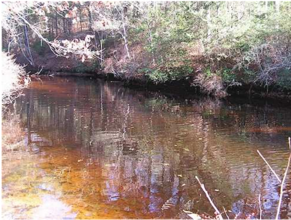
Upstream view of undercut east bank
